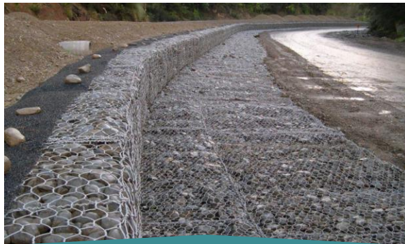
River Bank Protection
